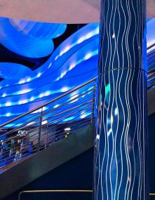
Designed to accommodate Georgia Aquarium's two million visitors per year, the columns are built to withstand high-traffic and heavy-duty cleaners, especially as more Americans resume indoor activities over the next year. Rolled from 0.090" solid-core aluminum and spanning more than 14 feet high, the columns are ready to support attendees while maintaining a good-as-new appearance.
