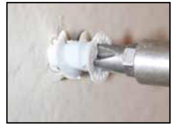
3 Set drywall anchor for screws if needed.
