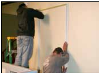
4 Anchor first Snap Bar and set second Bar parallel to the first and so on with the remaining Snap Bars.
