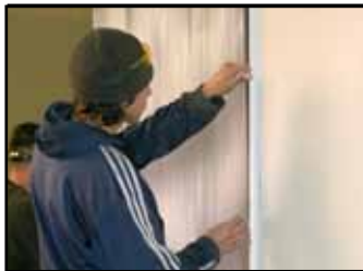
5 Position and snap panels into the Snap Bars starting with one corner.
