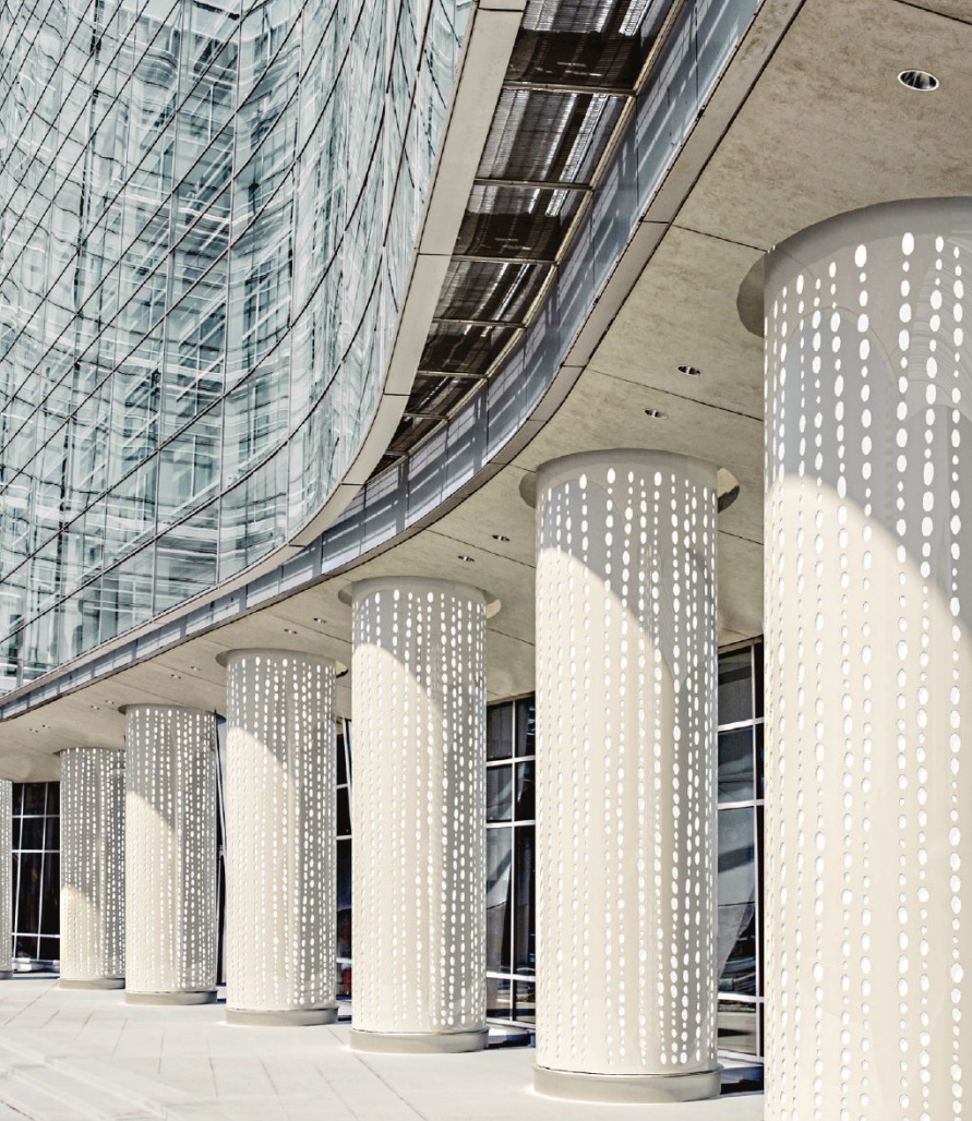
Architectural-grade vinyl finishes increase the longevity of metal columns.
