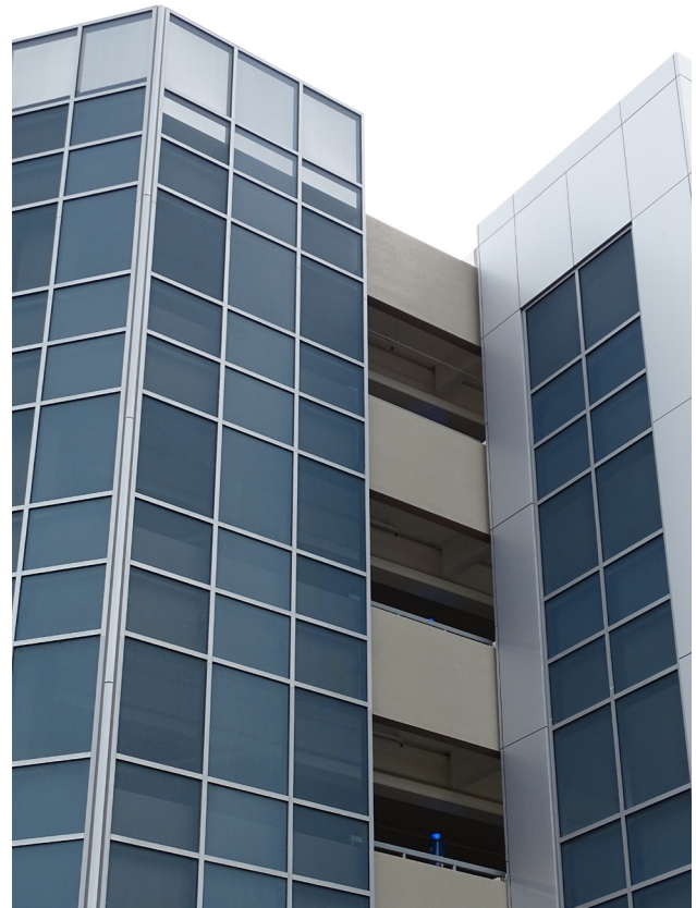
6-Level Gilead Sciences Parking Garage Foster City, CA
